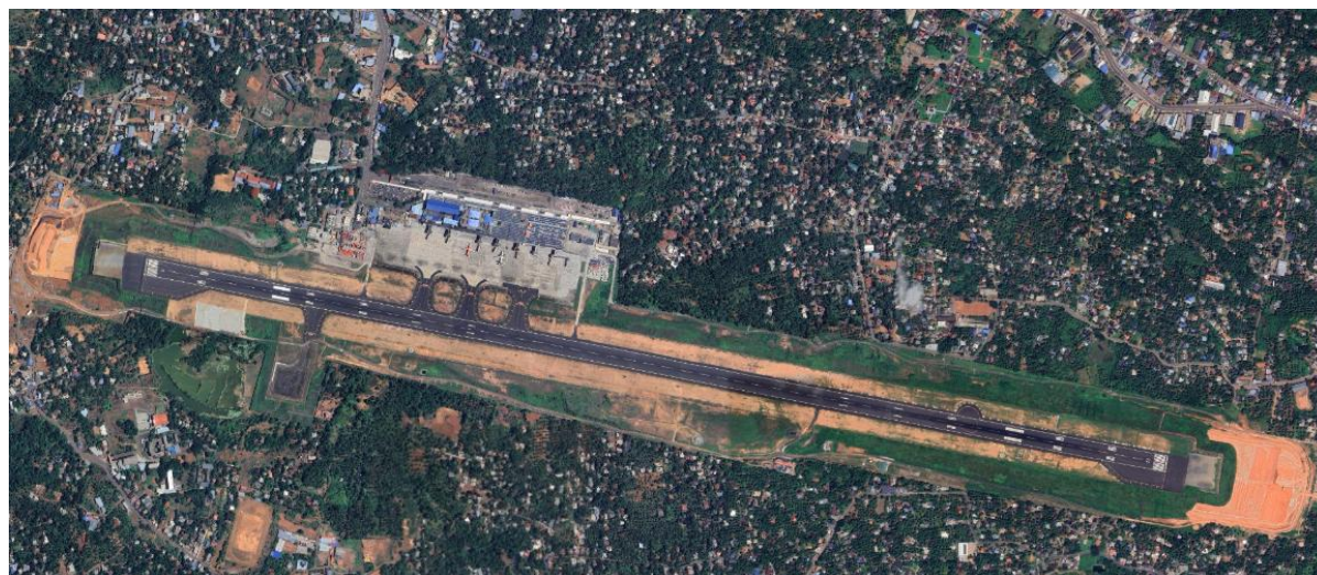
Figure 1: Satellite image of the work in progress of the RESA at Calicut International Airport
