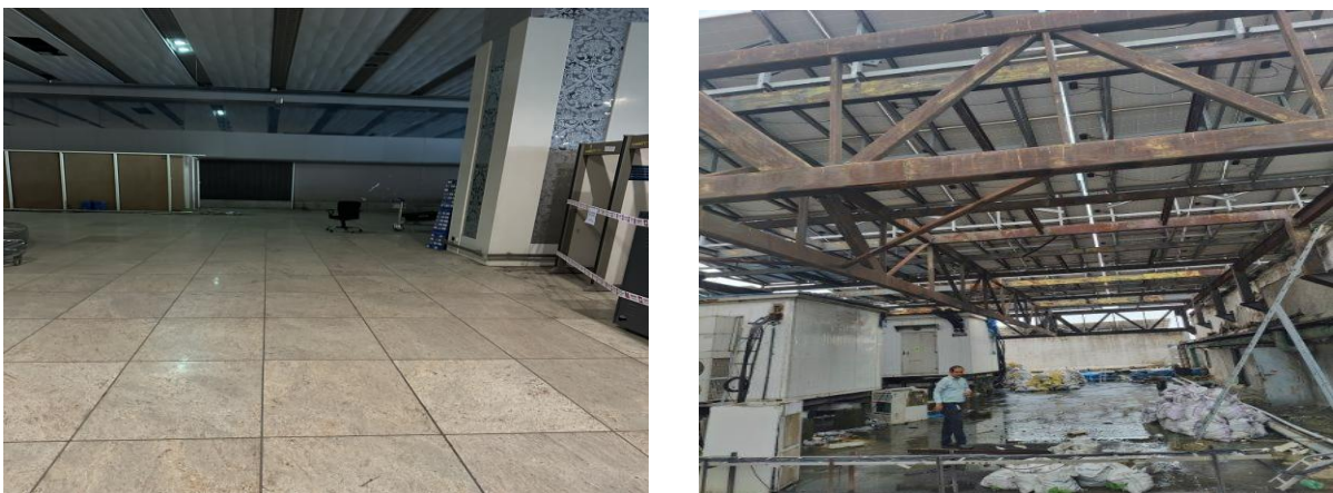
Figure 27 – T1 A – Arrival (GF), AHU (Terrace)
