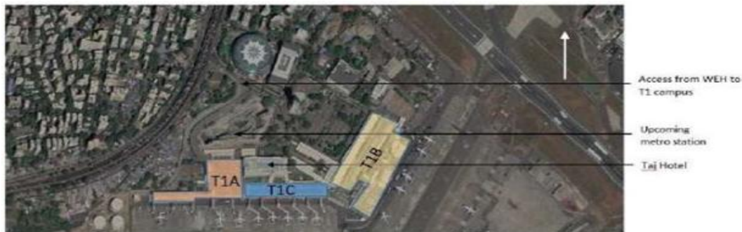
Figure 16 – Overview of the existing T1
