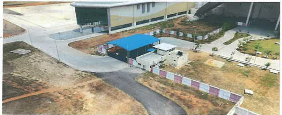
Compound wall, perimeter road, RCC drain for NITB
