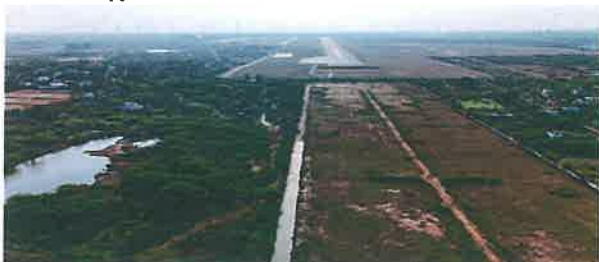
CAT - I Approach Perimeter Road
