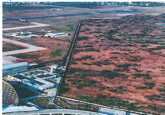
Operational Road Perimeter Road
