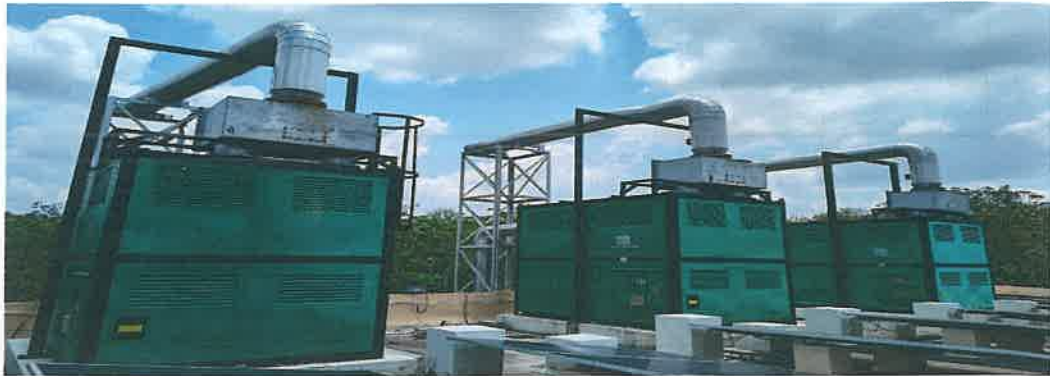
RETROFITTING EMISSION CONTROL DEVICE-1010 KVA DGSE – Rs. 0.88 Crores
