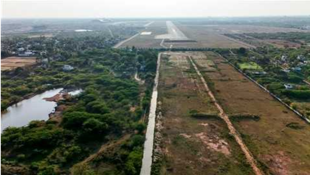
CAT - I Approach Perimeter Road
