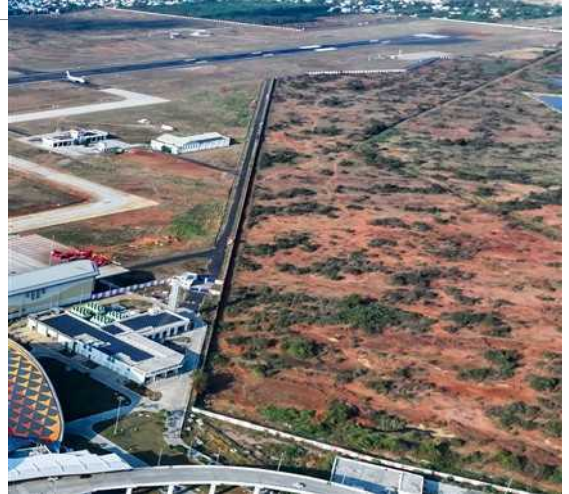
Operational Road Perimeter Road
