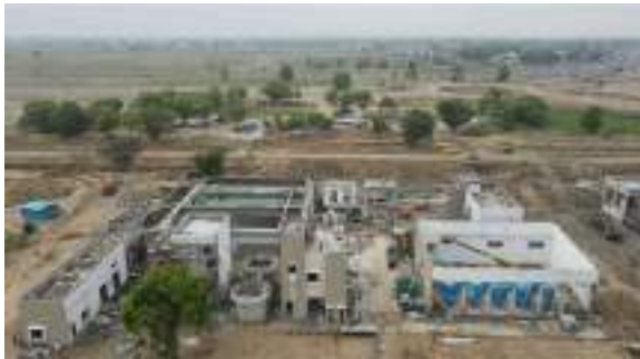
4.5 MLD STP under construction Aligned with Zero Liquid Discharge
