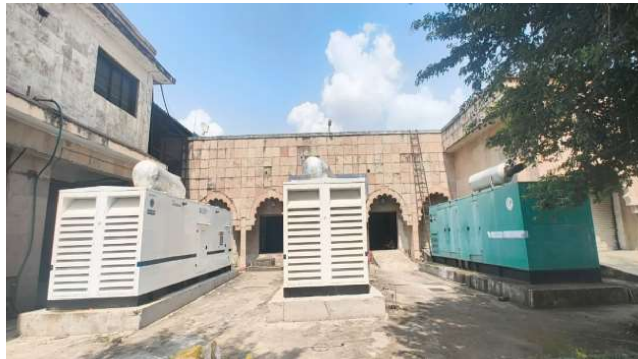
ONGOING ELECTRICAL WORK 1 – SITC of DG Sets
