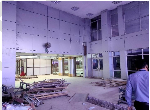
TERMINAL 3 UNDER RENOVATION WORK
