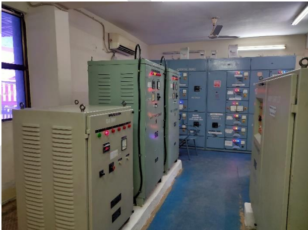
CONTROL PANEL AREA
