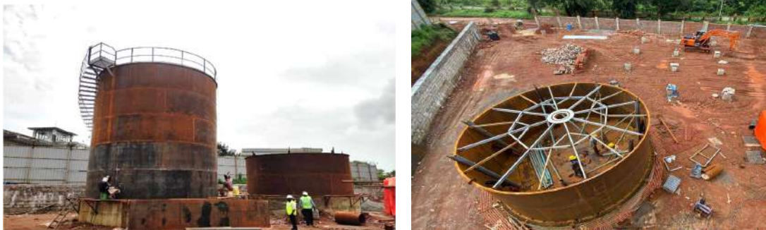
Progress photos of the construction of the Fuel Farm facility
