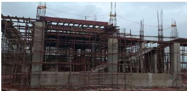
Progress photos of the construction of the Cargo facility
