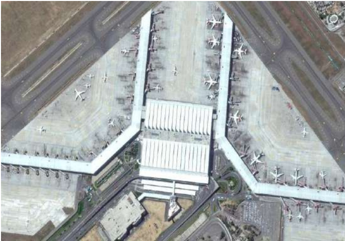
Delhi Airport Terminal-3
