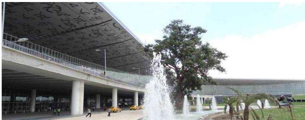
City-side view of new Terminal Building at Kolkata
