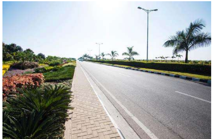
Landscaped approach road at Bangalore airport
