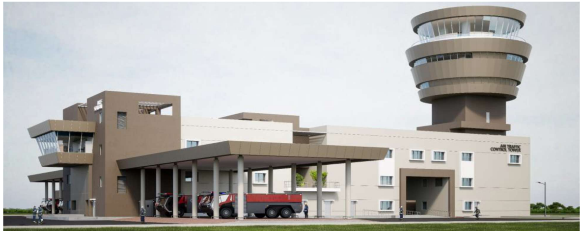
Figure 5: Airside Buildings – ATC and ARFF Tower
