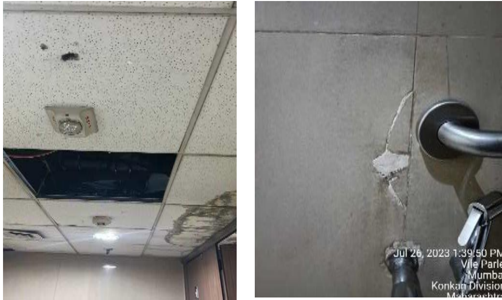
Figure: Existing condition of Washrooms at T2
