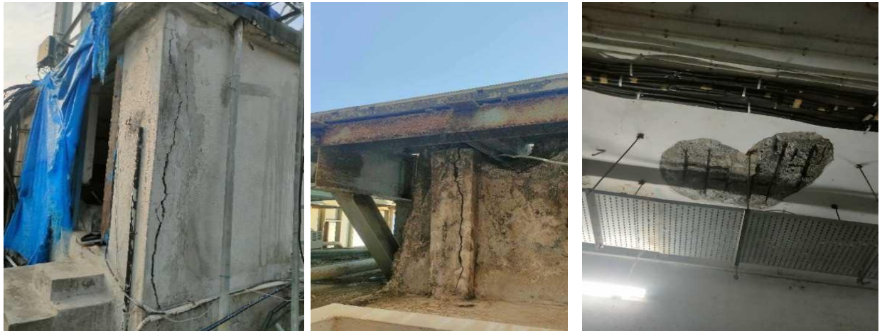
Figure: Existing structural damages in T1
