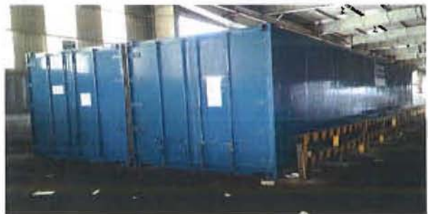
Dedicated storage facility for Pharmaceuticals (40' Containers – 04 No's)
