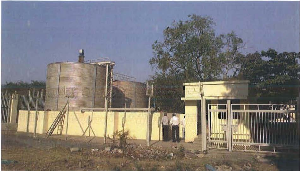
Sewage Treatment Plant for Cargo Services
