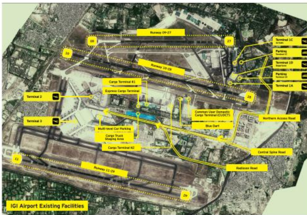
Figure 1: Image of Airport Facilities Pre-implementation of Phase 3A Expansion Project
