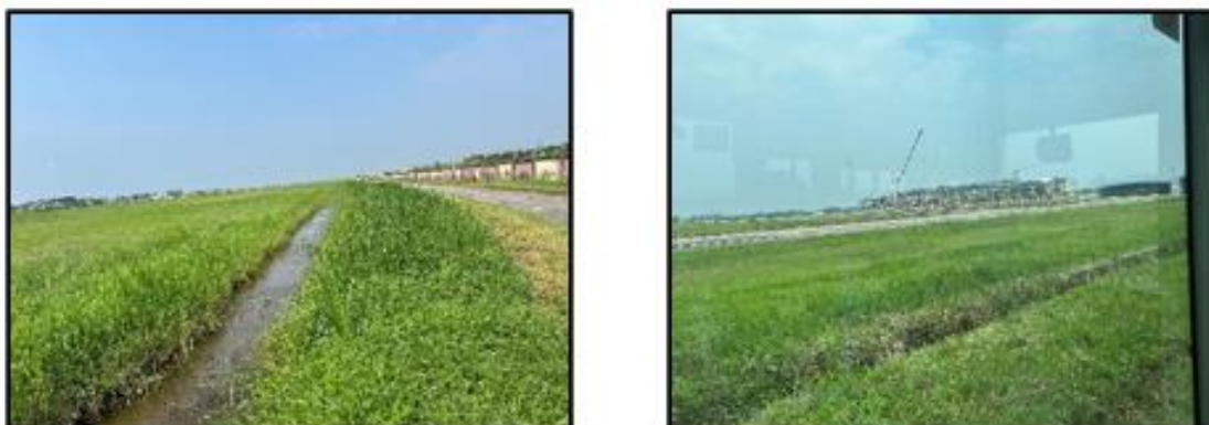
Figure 7: Existing drainage system at LGBIA
